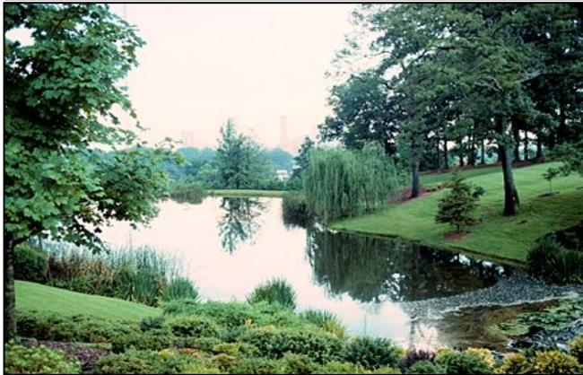
**Description:** A constructed water quality basin that has a permanent pool (or micropool). Runoff from each rain event is detained and treated in the pool primarily through settling and biological uptake mechanisms.
