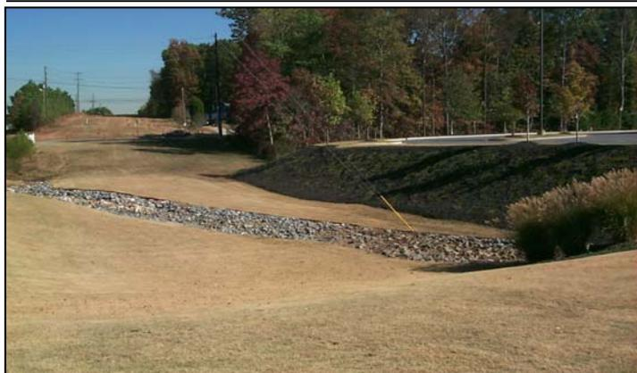
**Description:** A surface storage basin or facility designed to provide water quantity and quality control through detention of stormwater runoff.
