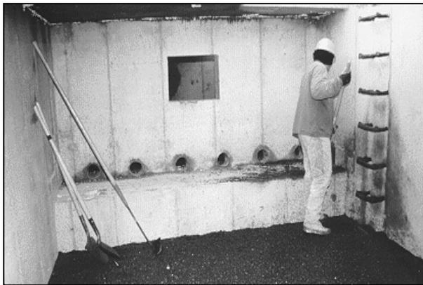
**Description:** The underground sand filter is a design variation of the surface sand filter, where the sand filter chambers and media are located in an underground vault.
