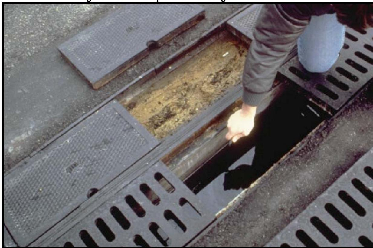
Multiple configurations have been developed for underground filters including the DC filter and the Delaware filter. The DC filter is intended to treat stormwater that is conveyed by a storm drain system. The Delaware filter (also known as the perimeter sand filter) is designed to collect flow directly from impervious surfaces and is well suited for installation along parking areas. Both systems operate in the same manner.
